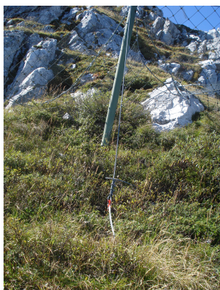
Fig. 5: example of a complete pulling out of a downhill anchor in a snow net
