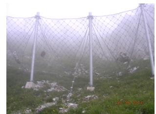
Fig. 3: example of the impact of rock blocks on snow nets
