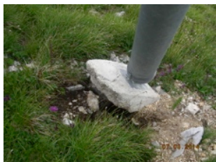
Fig. 7: example of downhill rotation and translation of the post foundation of snow nets
