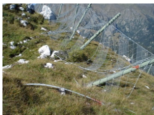
Fig. 4: example of a complete pulling out of an uphill anchor in a snow net
